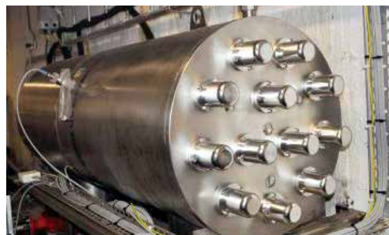
UV water purification systems installed at the water treatment plant.
