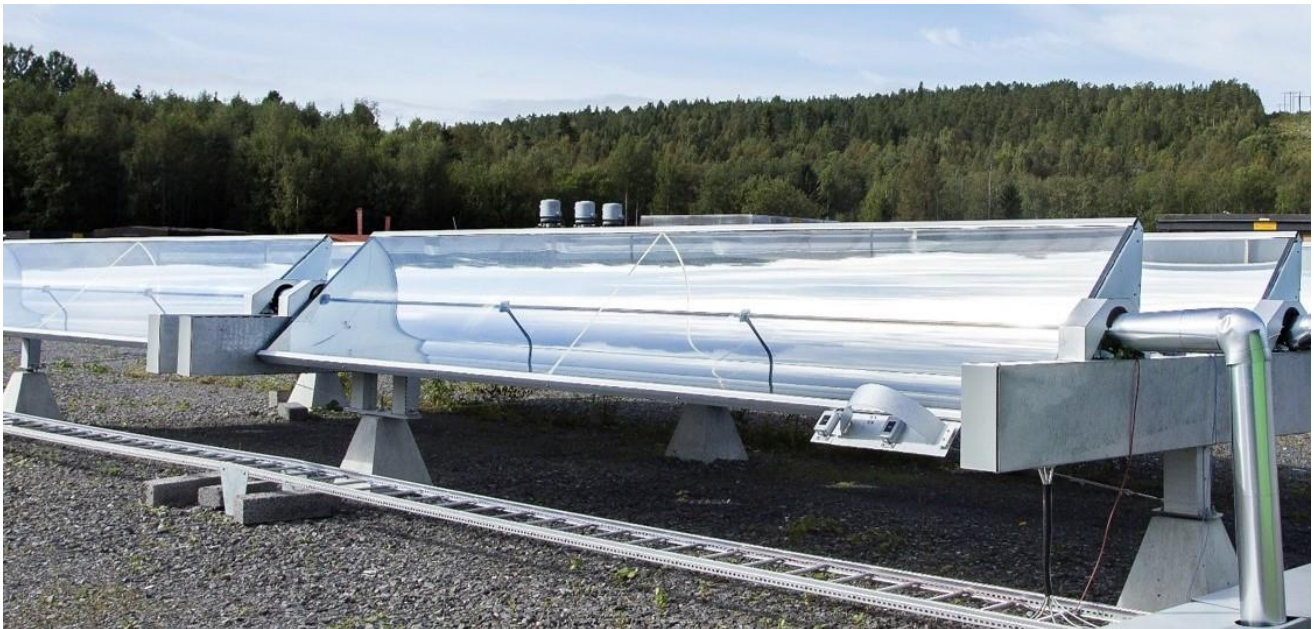
Figure 1. Field installation of the Absolicon T160.
